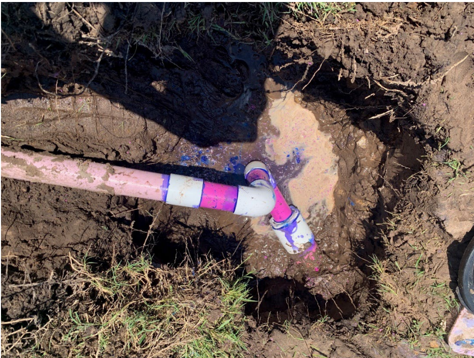
Repaired mainline on Waterset Blvd.
